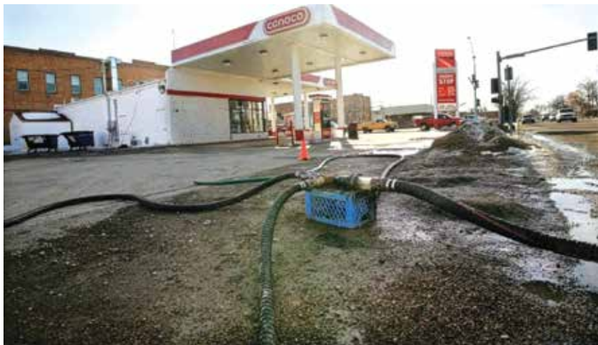
Gas station cleanup from Billings Gazette
